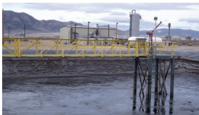
Liquid effluent is pumped from finishing barns to a one million gallon influent basin (above left). Submersible pumps transfer the liquid via a series of pump lift stations (above right) to the covered digesters.
