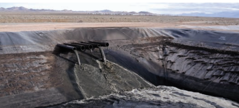
Liquid effluent is pumped from finishing barns to a one million gallon influent basin (above left). Submersible pumps transfer the liquid via a series of pump lift stations (above right) to the covered digesters.
