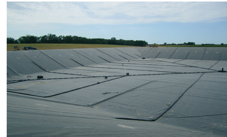
Completed anaerobic bio-gas collection cover. The wastewater flows into the basin under the air-tight cover. (For scale; note the worker in the upper left hand corner of basin.)
