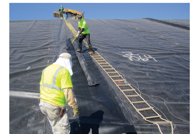
Installation crew meeting the challenge of a steep side slope dairy basin.
