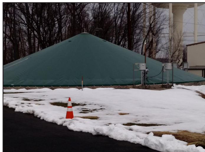
Winter 2018 -- IEC's Flexible Tank Cover system consists of a flexible geomembrane supported by a center column and tensioned with straps. Materials are high-strength, chemically-resistant, and UV-protected to ensure a maximum service-life under harsh conditions.
