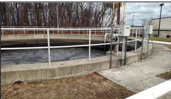
Prior to 2018, open equalization tank filled with septage (wastewater).
