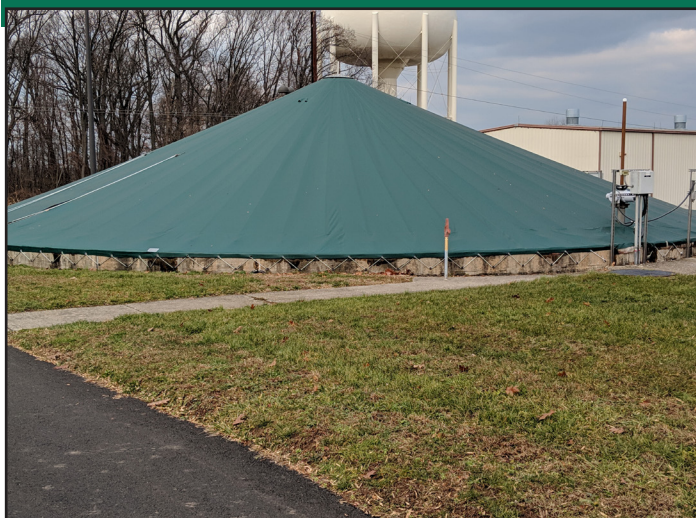
Fall 2018 – Newly installed Flexible Tank Cover system designed and installed by Industrial & Environmental Concepts, Inc. (IEC) for the NAWC Septage Treatment Facility (Warminster, PA).
