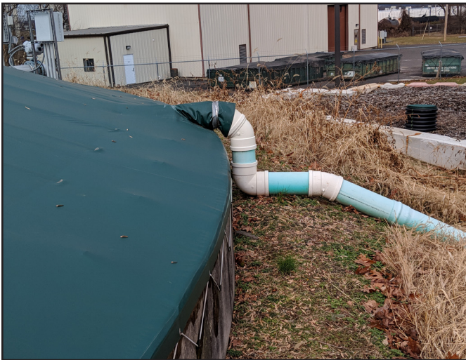
Biofilter draw-off connection to cover.
