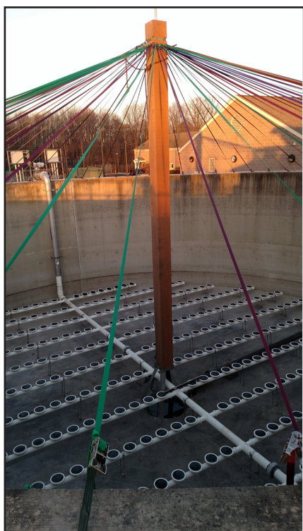
Center support column with radial tensioning straps.
